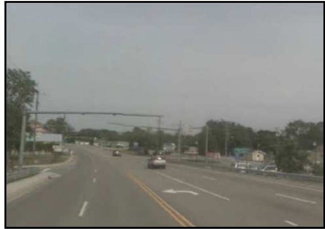
Existing US 64 in Tyrrell County
